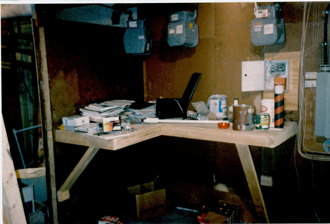
A-8 PHOTO OF THE BENCH I BUILT IN NOVEMBER OF '91. THIS WAS MADE OUT OF THE REMAINS OF THE WOOD USED TO MAKE THE BOXES FOR CSM. THE BOX WITH THE DOOR OPEN (RIGHT SIDE OF PHOTO) IS THE ALARM SYSTEM THAT WAS INSTALLED BY ME AND RICH BROWN ON THE FIRST OR SECOND OF NOVEMBER. THE PAINT CAN WAS THE REMAINS OF THE PAINT THAT CHRIS PUNIS USED TO PAINT THE OUTSIDE FRONT OF THE OFFICE.
