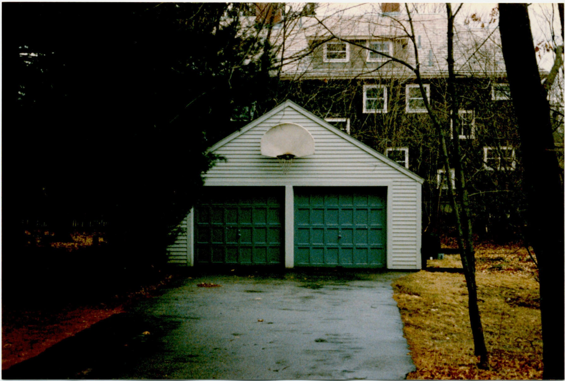
W-5 PHOTO OF GARARGE, FRONT VIEW
